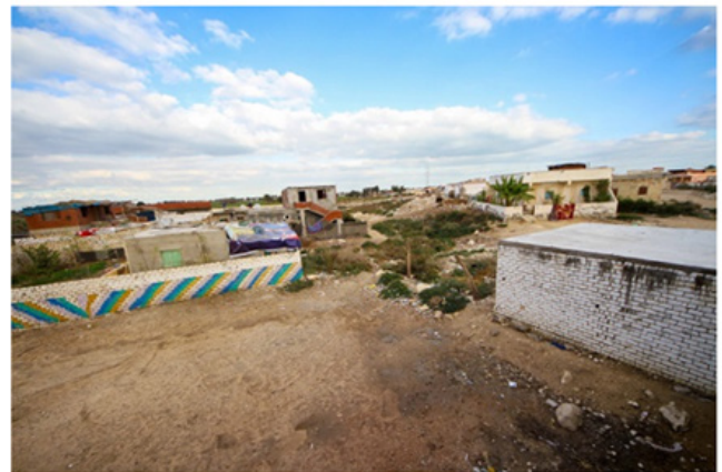
Figure 6: Naga Oun before improvement project.
