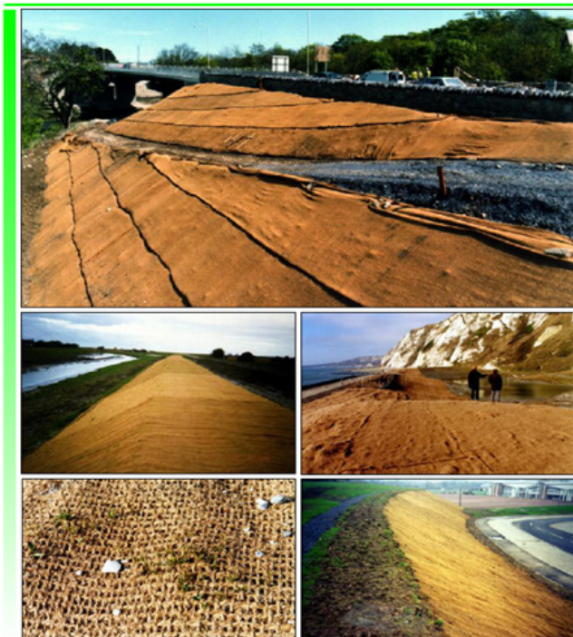
Figure 2: Coir mesh used in Erosion Control Measures [32].
