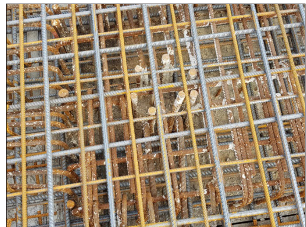
Figure 3: Picture of a finely meshed reinforcement network for watertight concrete constructions.
