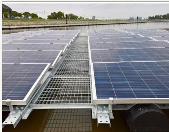
Figure 1: Detail of our floating platform on tengeh reservoir (Singapore).
