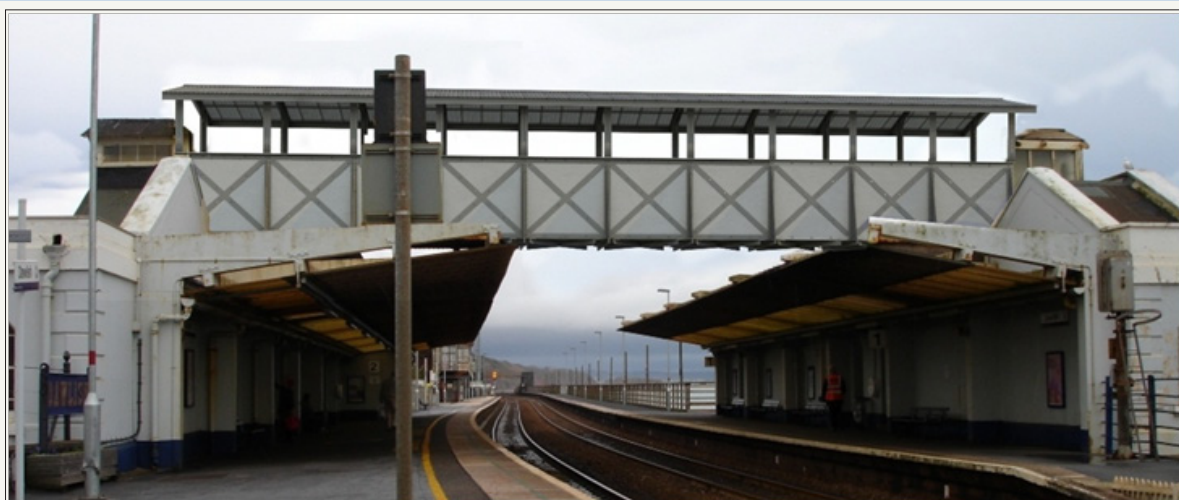
Figure 1: Dawlish footbridge, Exeter, United Kingdom [2].
