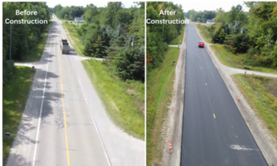
Figure 3: Pavement condition before and after construction.
