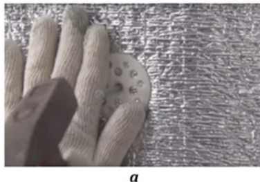
Figure 1: Formation of a seamless shell: a - mechanical fastening of the insulation sheet; b - welding of joints of rolled polyethylene foam.
