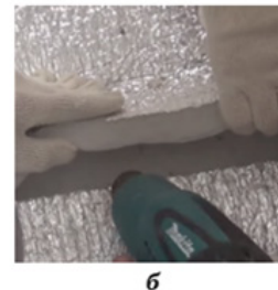
Figure 1: Formation of a seamless shell: a - mechanical fastening of the insulation sheet; b - welding of joints of rolled polyethylene foam.
