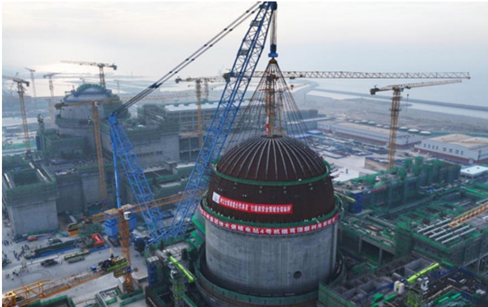
Figure 3: On-site of the dome hoisting operation of unit 4 of xudapu nuclear power plant (a Sino Russian cooperative project).
