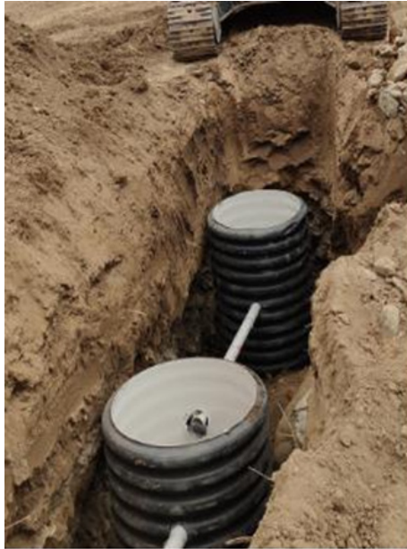
Figure 11: Straight cylinder type buried observation in Machu, Gansu Province.
