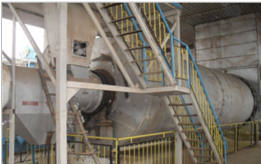
Figure 2: General view of the drum dryer 2CB-10.
