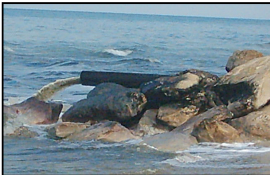
Figure 3: Discharge of untreated or partially treated wastewater into the Mediterranean Sea via multiple coastal outfalls along the Gaza Strip coastline.
