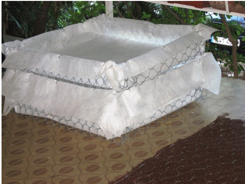
Figure 3: Setting on the ground of "Reno" mattress.
