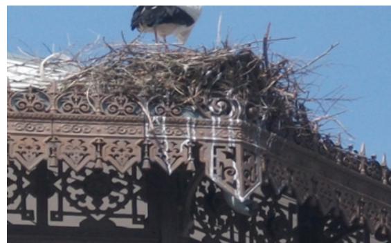
Figure 4: Remains of excrement, under a stork's nest built on the roof of the banstand in the Plaza de Cervantes in Alcalá de Henares (Spain).
