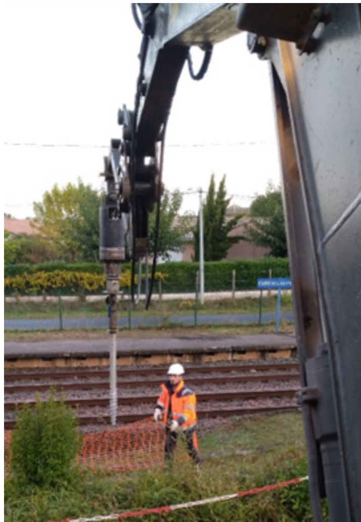
Figure 7: Ground screw GEOVIS before installation..
