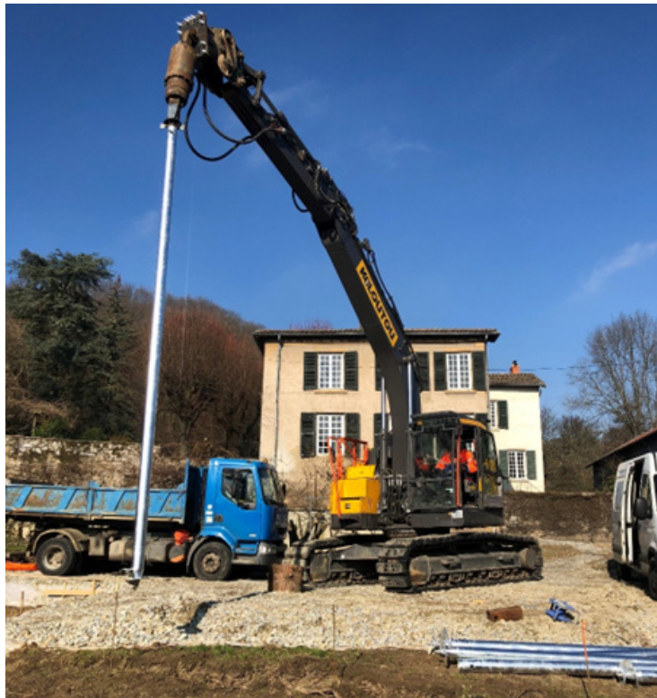
Figure 2: Installation of ground screws using a 20 tons excavator.
