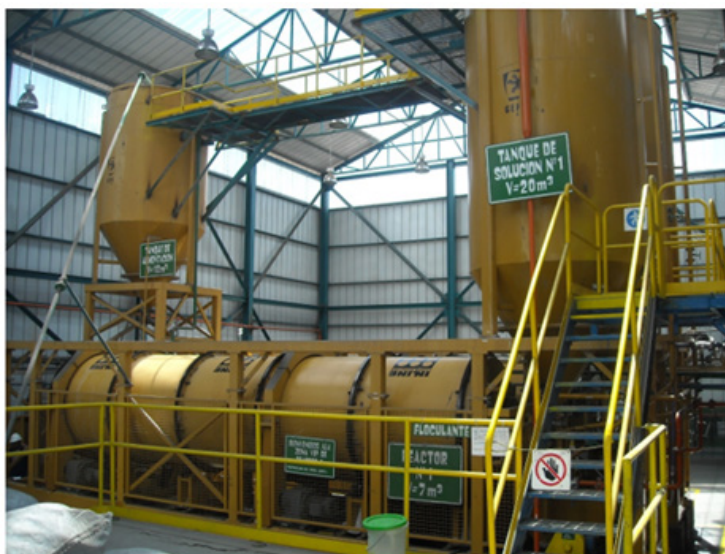
Figure 4: Photograph of the ILR 5000 reactor, with the feed tank and the 20m 3 solid/liquid separation tank.
