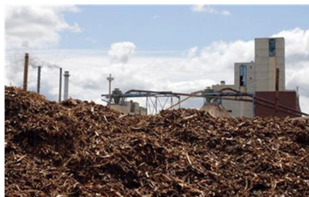
Figure 1: Photo of biomass powder clustering before introduced into boilers/furnaces.
