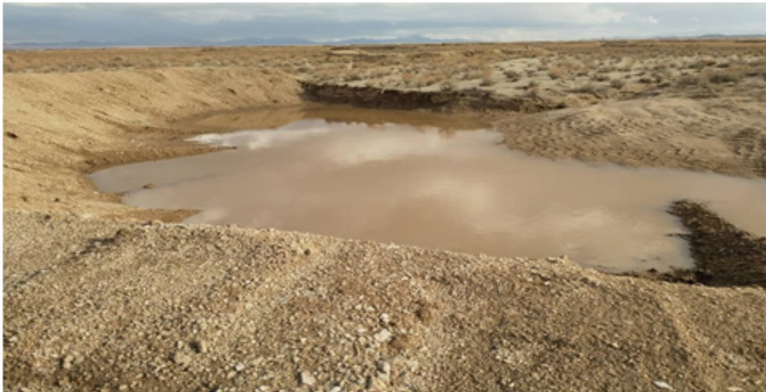
Figure 7: An Arc Percolation Tank (APT) structure in the Chahderaz plain.
