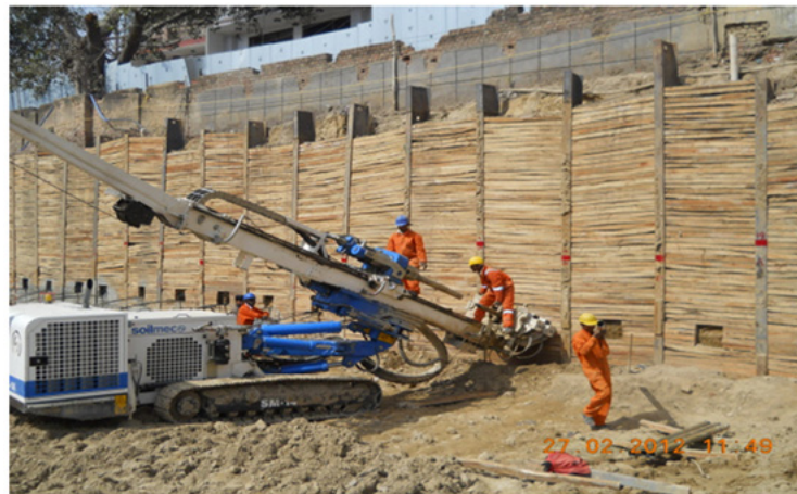
Figure 1: Soldier pile with timber lagging and installation of ground anchored.
