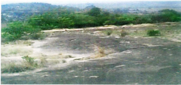
Figure 6: Cracks and fissures on Rock A.
