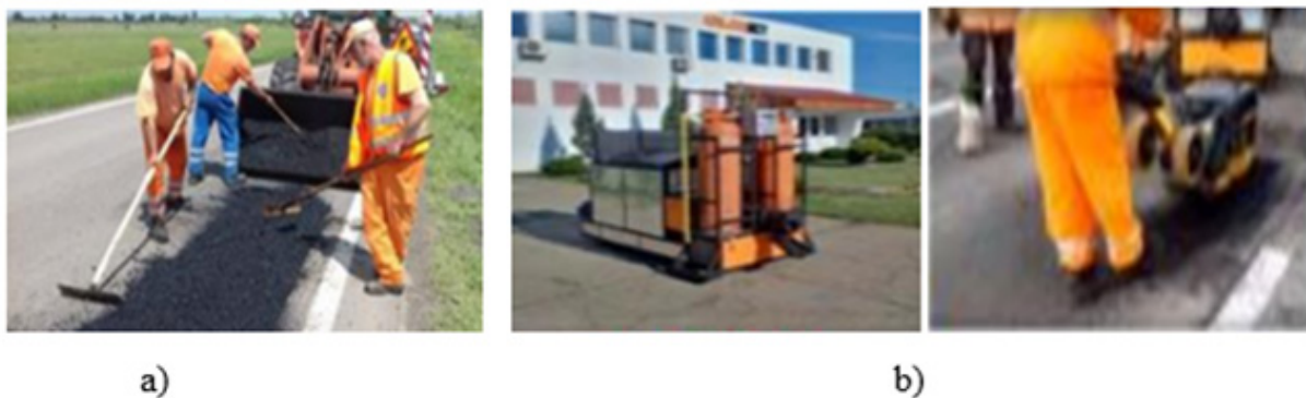
Figure 2: Wear layer repair operation (classic - a, with IR technology- b).
