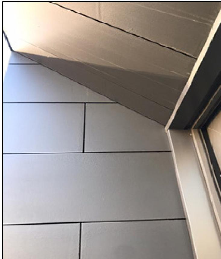
**Figure 2:** The house exterior after 5 years (close up view of the aluminum coating).
