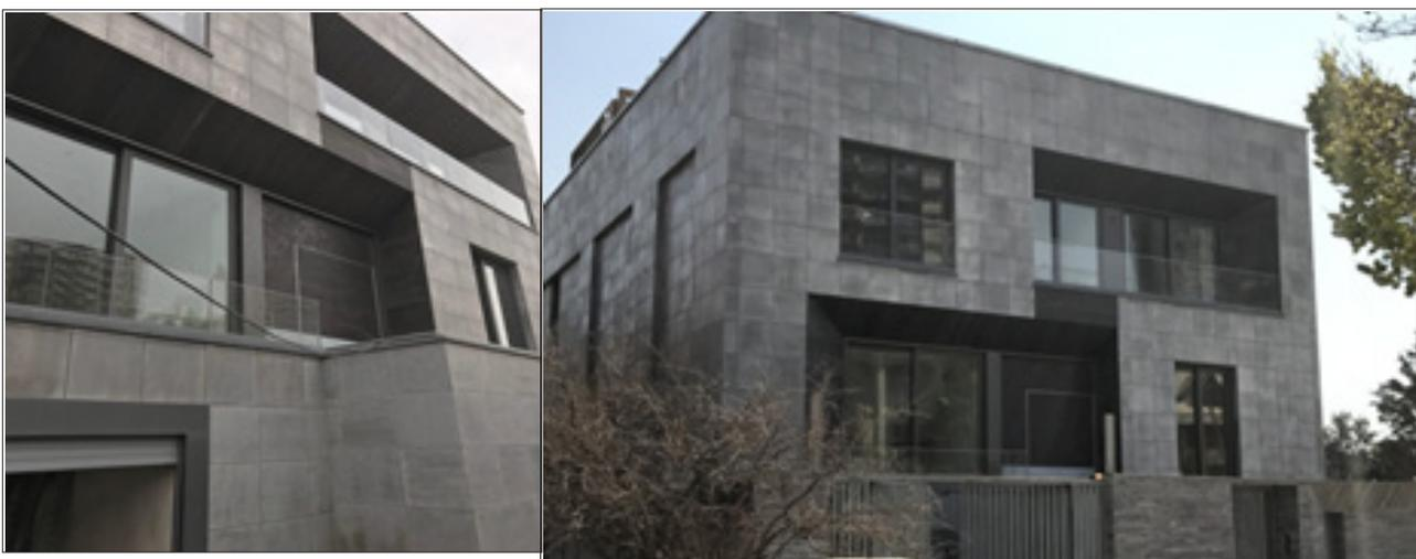
**Figure 1:** The house exterior with the ceramic tiles coated by Aluminum (light color) and German silver (dark color) right after installation (Left) and after 5 years (Right).
