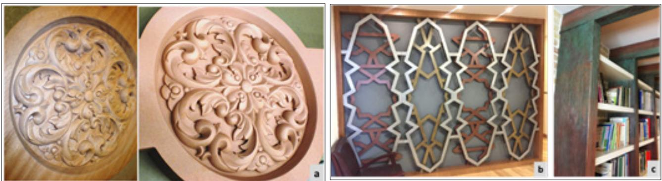
**Figure 3:** Examples of metal coated interior installations. Curved mahogany before and after copper coating (a), MDF installation with different metal coatings (b) and painted copper coating on wood beams (c).
