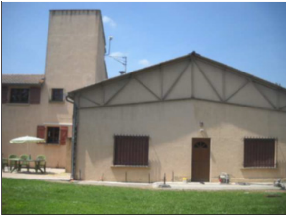
Figure 4: General view of the studied site.
