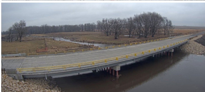
Figure 2: Buffalo Creek bridge built in Iowa in 2018 used over 100 tons of CGR for deck, abutments and parapets [1].
