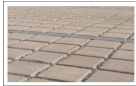
Figure 5: Permeable paving ( https://www.pacificpavingstone.com ).
