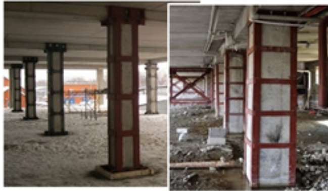
Figure 9: Strengthening of columns of multi-storey buildings.
