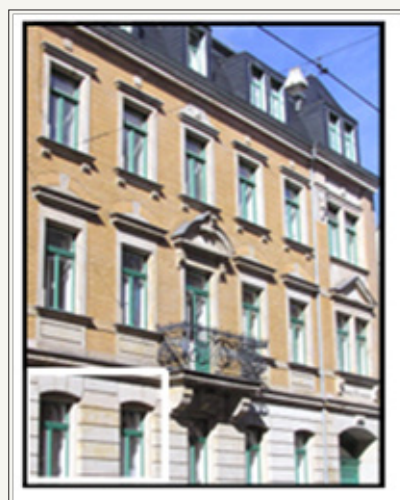
Figure 6: Gründerzeithaus in Dresden, energetical renovation of the wall in view.
