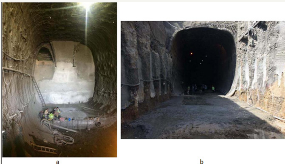
Figure 3: Modares tunnel initial lining a) inside view b) outside view.
