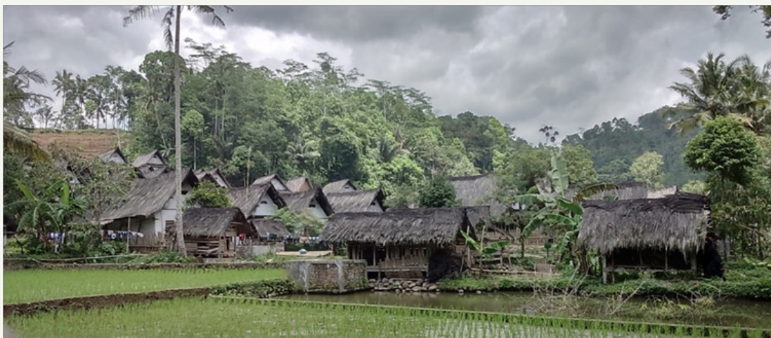
Figure 1: Houses in a village in Indonesia using roofs made from sugar palm fibres.
