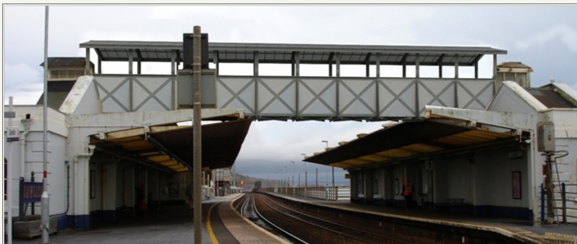
Figure 1: Dawlish footbridge, Exeter, United Kingdom [2].
