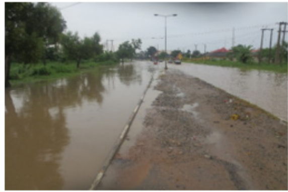
Plate 2: Flood site along Eniong Street
