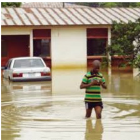
Plate 3: Destruction of Buildings by Flood along Atiku.
