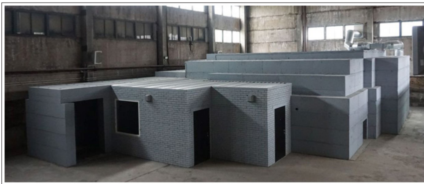
Figure 1: Concrete shielding with a GAA demo-testing facility inside an industrial hangar.
