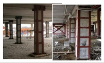
Figure 9: Strengthening of columns of multi-storey buildings.
